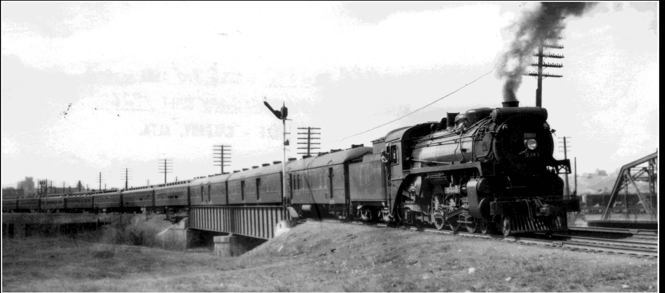
Bridge over the Elbow River a two span HDPG was installed with the double track in 1911. It will be replaced with a ballasted deck span in 1985.
