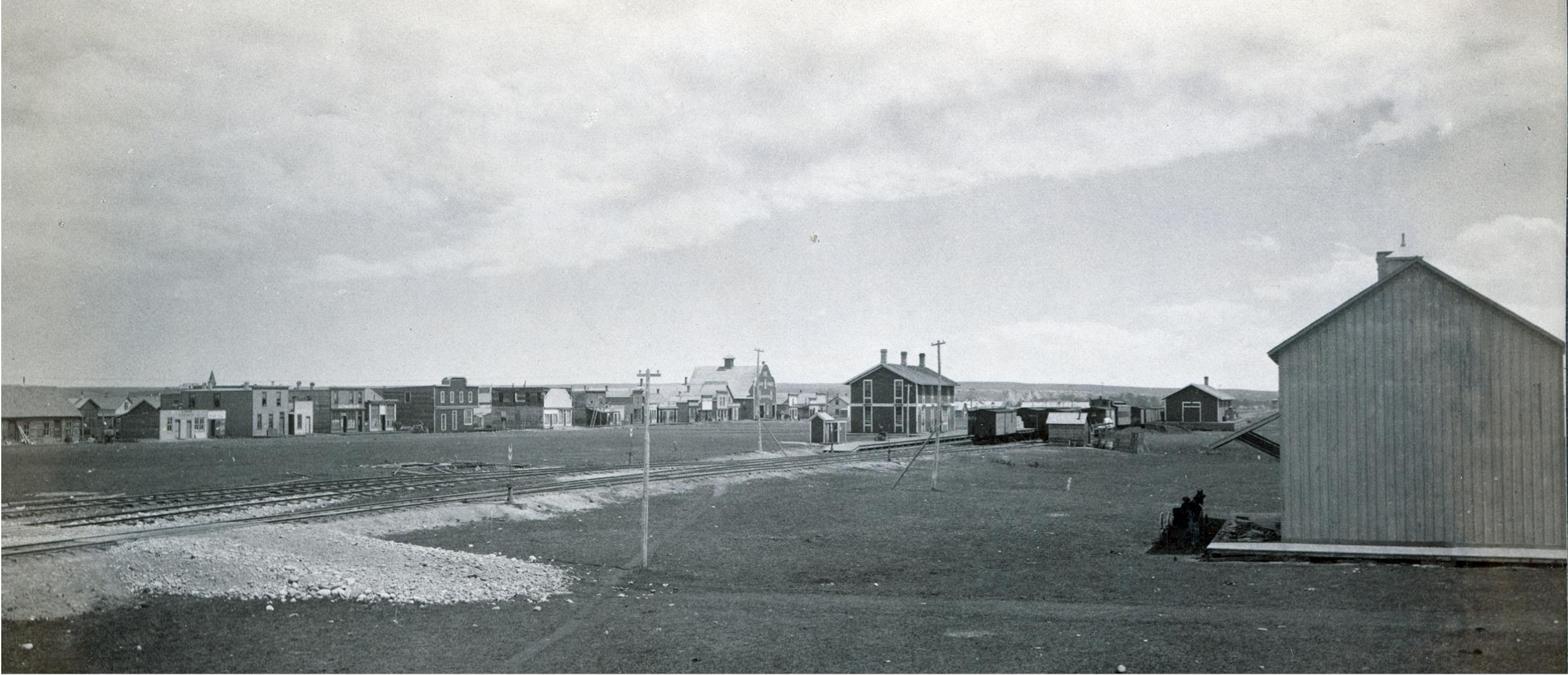
New station 2 nd was completed in February 1884.
