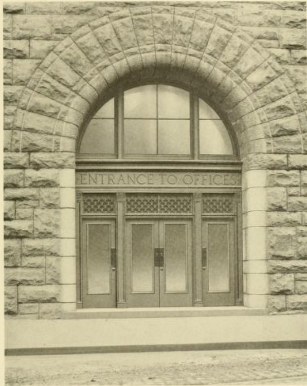
Windsor Station, Montreal Cast Iron Office Entrance (Hollow Steel Doors) Barott, Blackader & Webster, Architect
